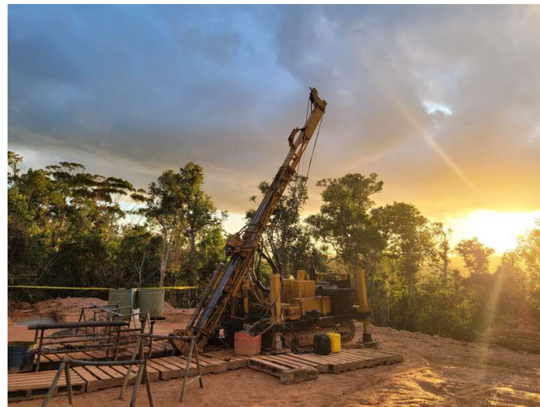
One of two Kalo Gold owned track mounted diamond drill rigs.
